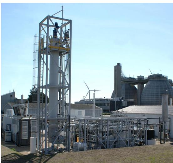
Fig. 1: Biomethanation reactor using CO<sub>2</sub> produced in the digesters to perform biogas-upgrading for gas grid injection
