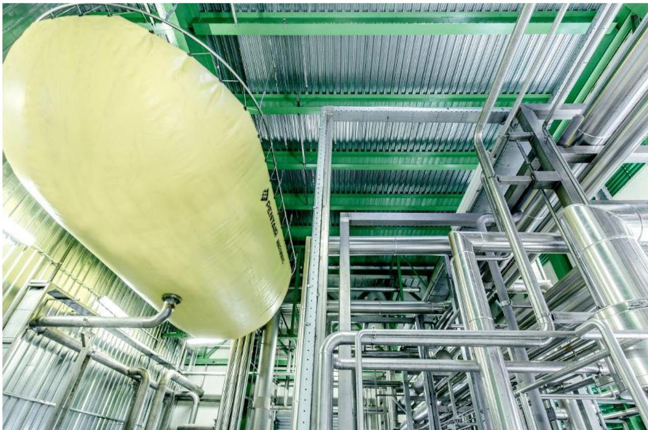
**Figure 18 - Example of gas balloon used for temporary storage**
