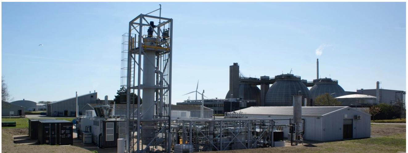
Figure 5 - View of the BioCat plant showing the reactor (left), balance of plant (center) and the biogas plant (background)
