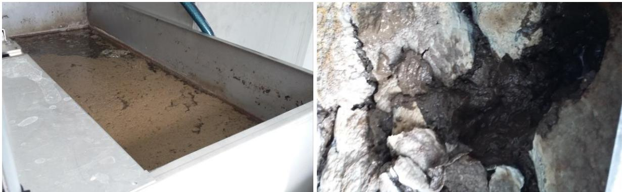
**Figure 75: Different stages in the formation of sludge layer in the flocculation tank**
