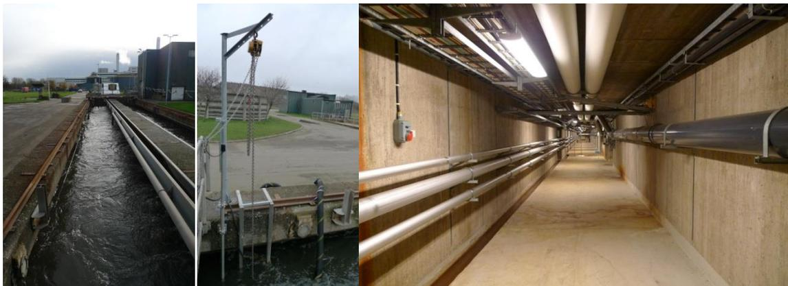
Figure 46: Grit chamber effluent (left), Crane for influent pump and influent turbidity sensor in the middle and pipe work towards the Discfilter plant (right)
