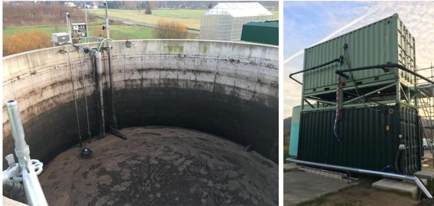
**Figure 8: Sludge storage tank and piping connections at the Westewitz WWTP**
