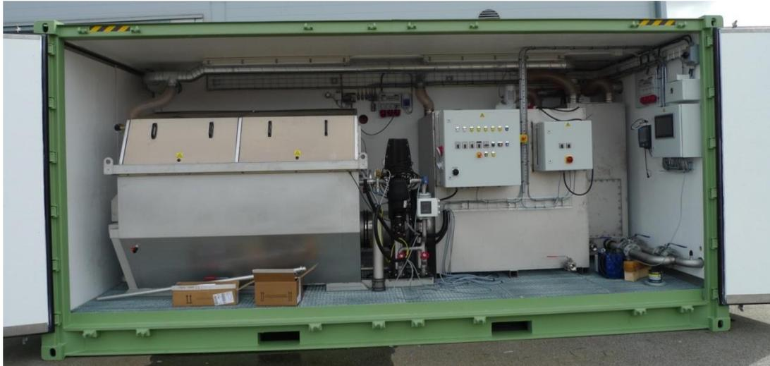
**Figure 6: The filter container at Westewitz WWTP, with coagulation tank, flocculation tank, drumfilter and control cabinets.**
