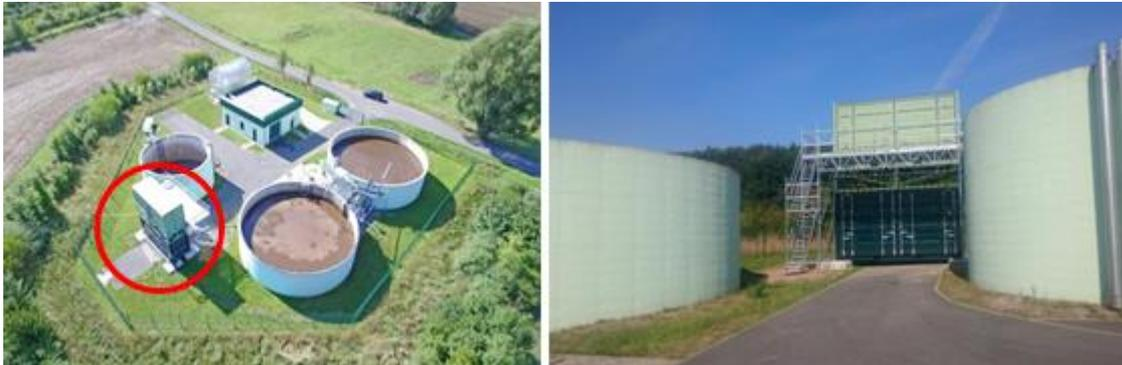
Figure 4: Left: Aerial image of the WWTP Westewitz after installation of the filtration plant (encircled in red); right: Front view of the containers of the filtrations plant located between the SBRs.
